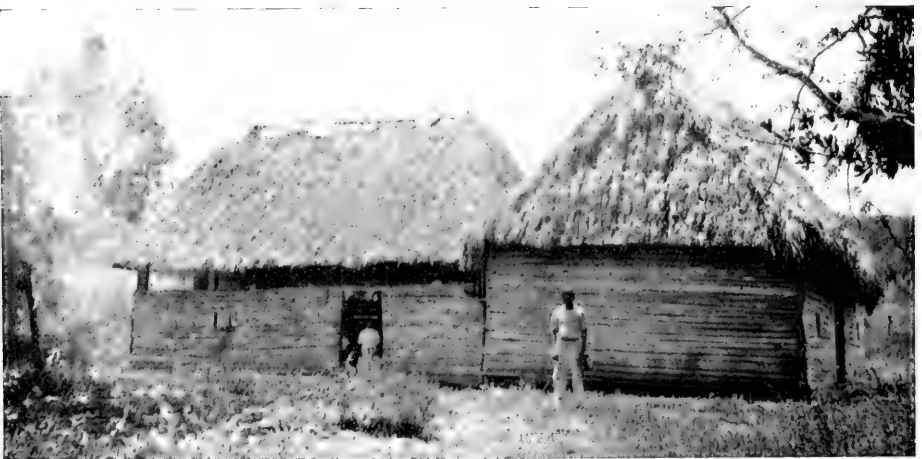
Casa de Suarez , the home of our mountain host. Country homes are made entirely from the royal palm; the trunk makes the walls of the house, the leaves make the thatched roof and the bracts cover the ridge pole. Stoves are uncommon, food is cooked over an open fire or on an earth-covered table
